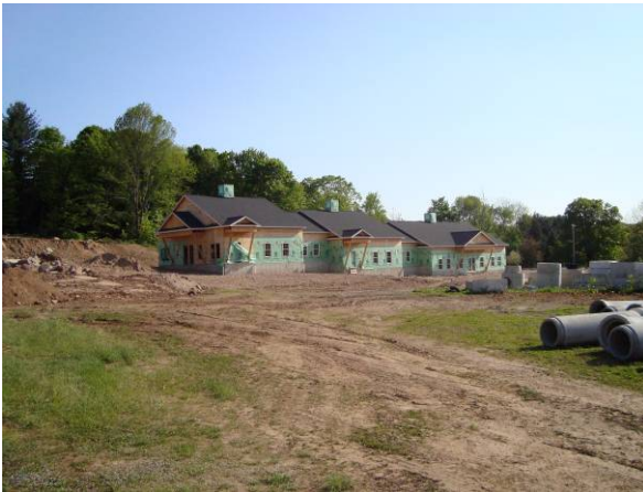
New Construction in the MQ District
